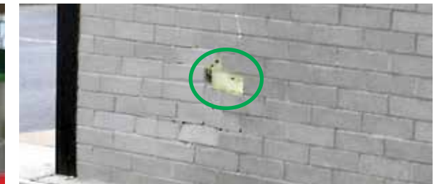
Photo 11.2 generally free of damage
