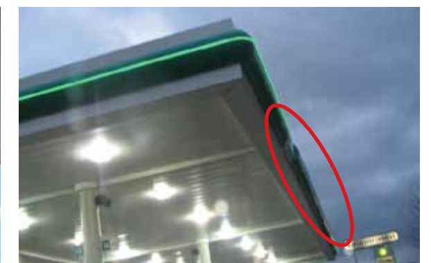
Photo 6.5 more than one 10 ft. section out
