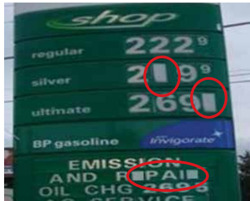
Photo 1.3 • missing numbers in pricing section • missing letters in reader board section
