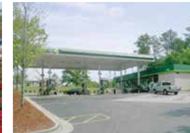
Photo 8.2 pavement area free of trash/debris
