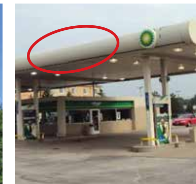
Photo 23.5 bullnose missing
