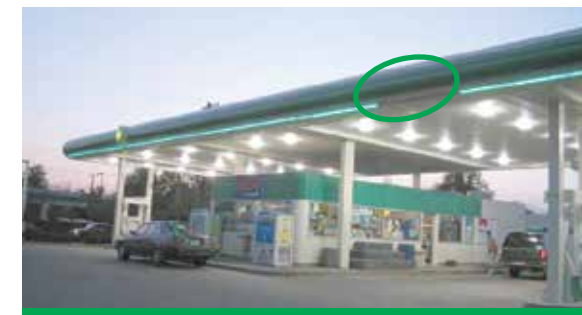
Photo 6.3 only one 10 ft. section out, all deck light functioning
