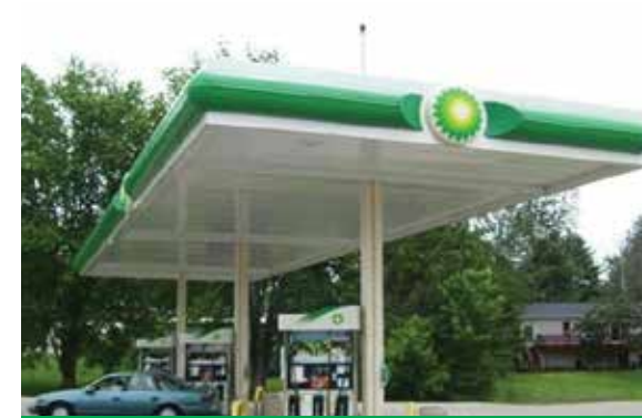
Photo 3.1 generally well maintained canopy deck, lights, columns and fascia
