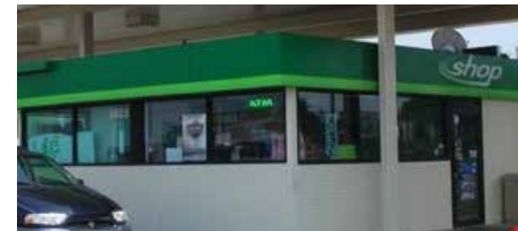
Photo 11.1 building exterior free of damage
