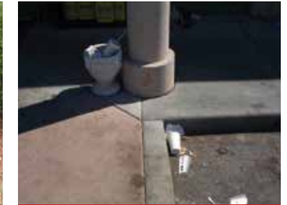
Photo 8.6 paved area accumulated trash/debris
